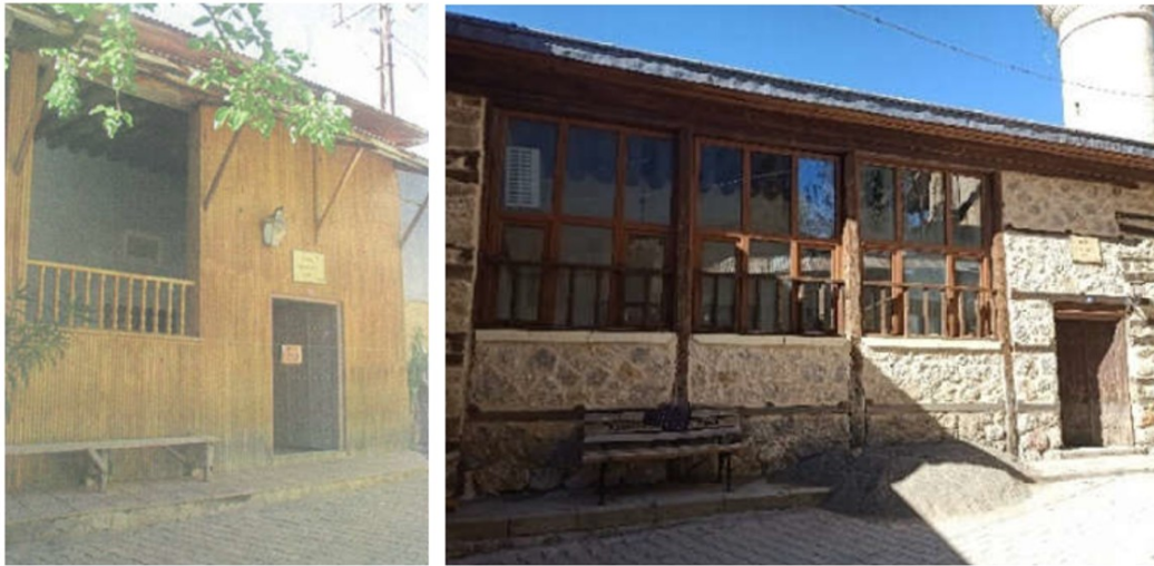
Figure 16. Son cemaat mahali of Bahçe Mahallesi Mosque, originally designed as a semi-open space but later enclosed through interventions and transformed into an interior space (left, [41]; right, author's archive)
