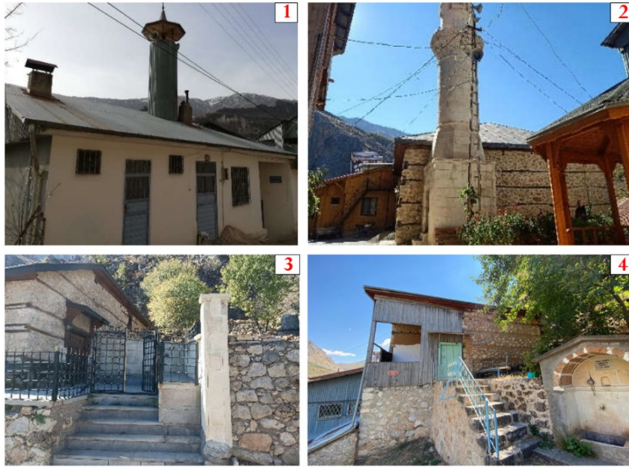
Figure 12. Structures and spatial elements located in the immediate surroundings of the mosques: (1) Lodging unit adjacent to Hacı Emin Efendi Masjid; (2) Built environment surrounding Bahçe Mahallesi Mosque; (3) Entrance area and adjacent hazire (graveyard) of Taşdibi Mosque; (4) Fountain and associated structures located around Kurtoğlu Mosque (by the authors)
